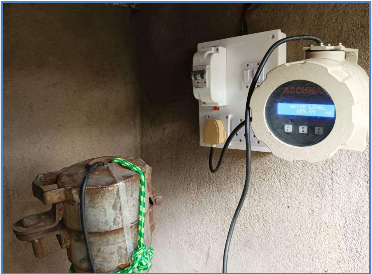
Picture 12 – Piezometer well
