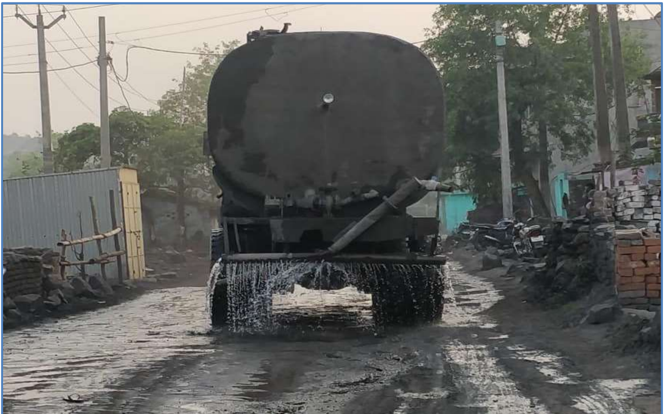
Picture 2 – Water Sprinkling on Transportation Road
